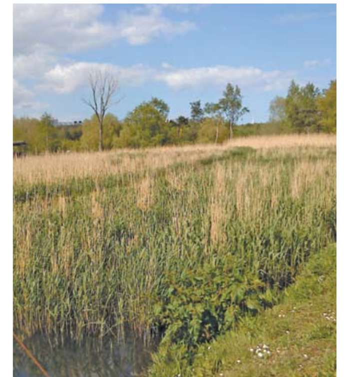
WWT Washington overland beds treating water entering the centre which originates from a sewage treatment works WWT
