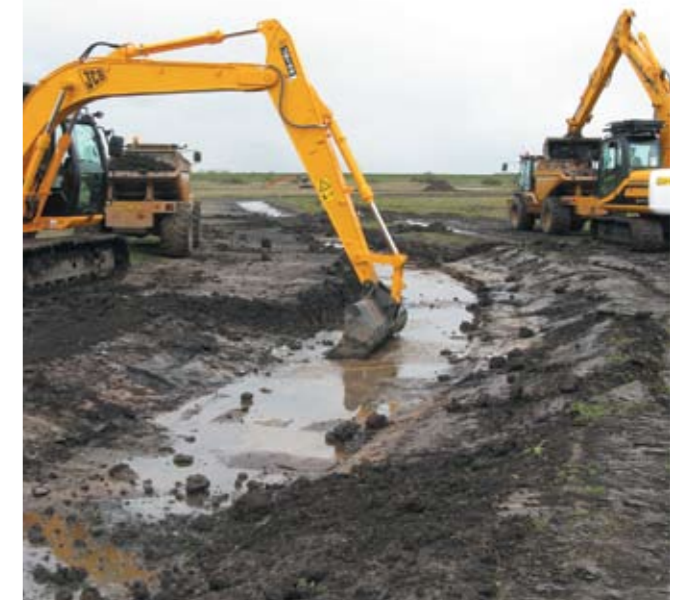
Excavating the central ditch for Lady Fen 2008
