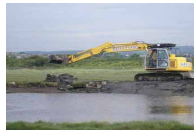
Excavator reforms banks to ensure water is held back in the lagoons following high tides. Nigel Williams/WWT.
