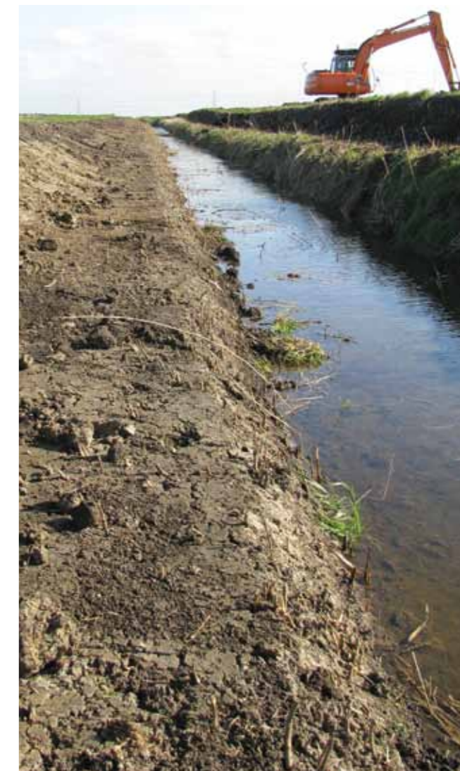
Creating shelves in ditches at Bank Farm. Leigh Marshall/WWT.
