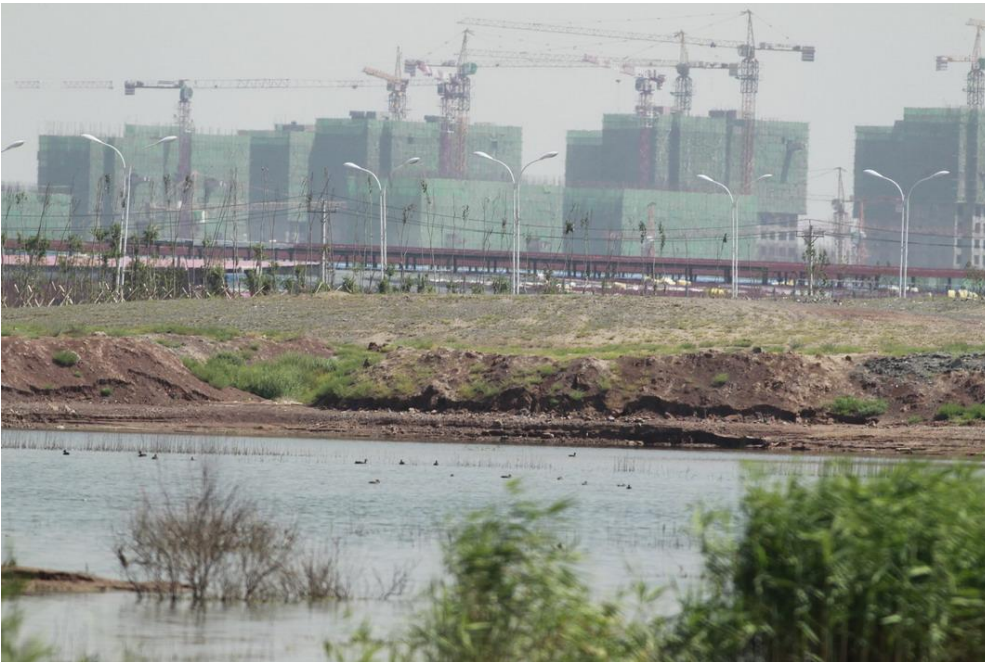
High-rise buildings being constructed near Bainiaohu, Urumqi, China (Ming Ma).
