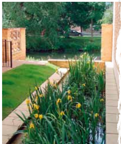
Riverside Court, Stamford – a canal as the final link in the management train, beginning with permeable paving, providing storage, amenity and biodiversity next to the River Welland. Photo: Bob Bray
