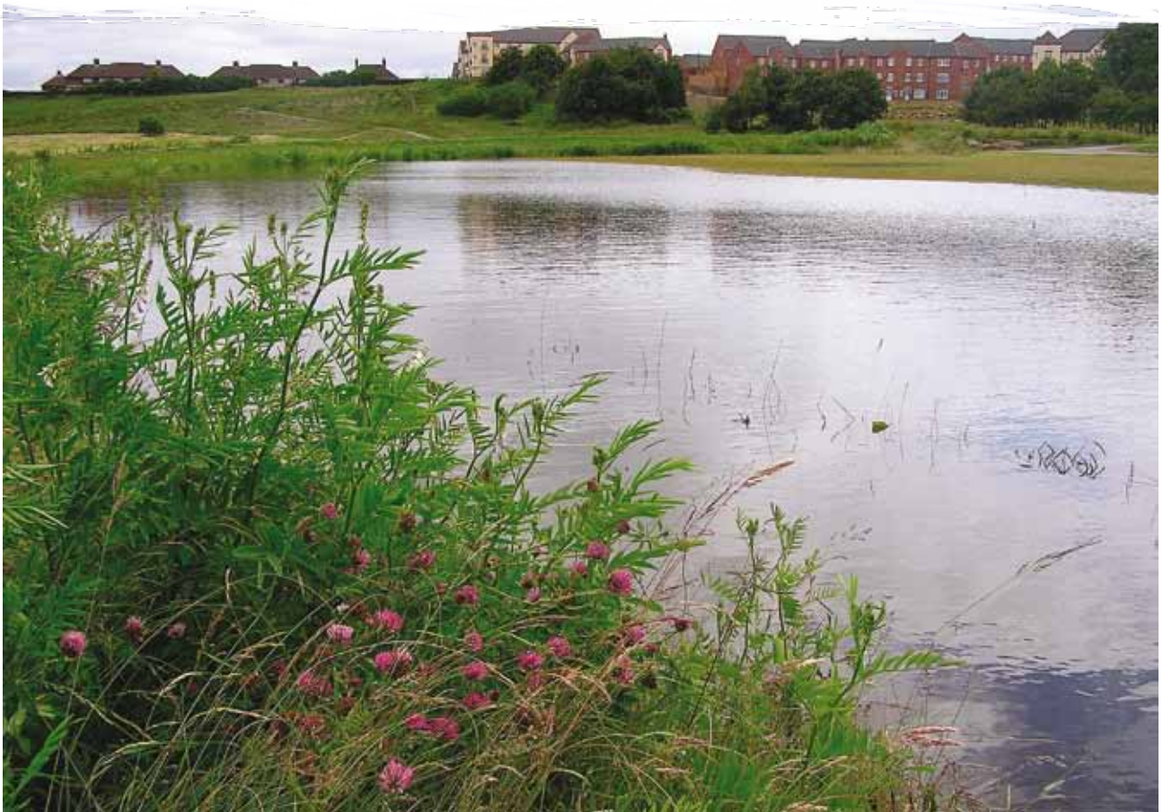
Manor Park Sheffield – under-drained sports and playing fields, the 1 in 100 year storage feature, two-thirds full at the beginning of the week in the 2007 floods but with football played on the Friday – a multi-use amenity space. Photo: Roger Nowell
