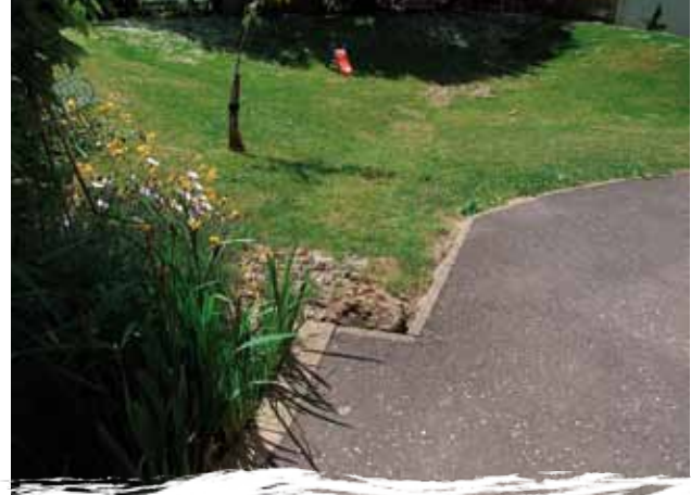
Springhill Housing, Stroud – a multi-functional detention basin and play space at the end of the management train that only fills after heavy rain. Photo: John Day (rspb)
