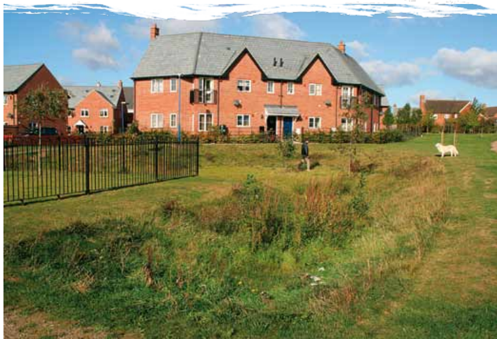
Lamb Drove, Cambourne – an open basin for occasional storage linked to a wet swale which is cut annually to enhance habitat whilst maintaining conveyance function. Photo: Bob Bray
