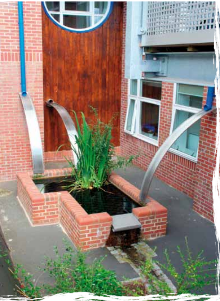
Fort Royal Primary School, Worcester – three rain slides deliver roof water into a raised pool which overflows into a set channel and rill before flowing to a wildlife pond in green space, all accessible by children. Photo: Bob Bray
