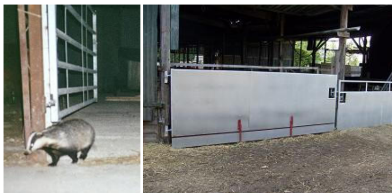
A badger entering a cattle shed, and a badger-proofed shed, which is a relatively straightforward means by which contact between livestock and wildlife can be reduced ( Fera ).
