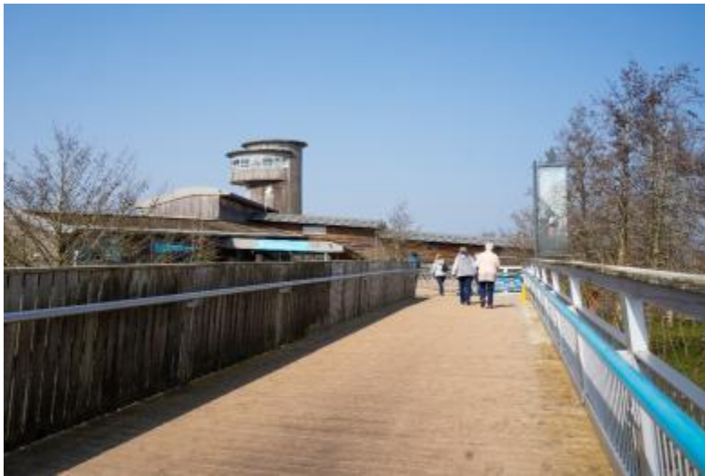
Ramp to the main entrance of the visitor centre.
