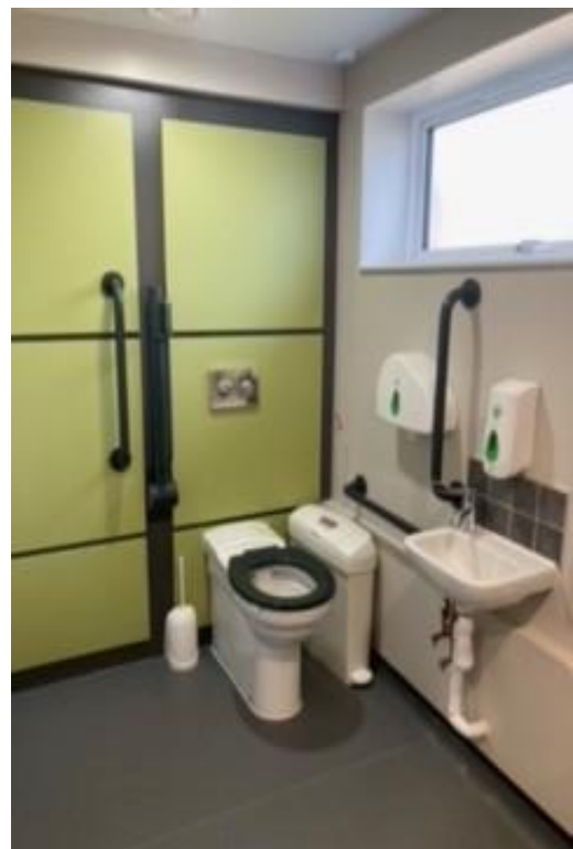
Toilet facilities in the Garden Room
