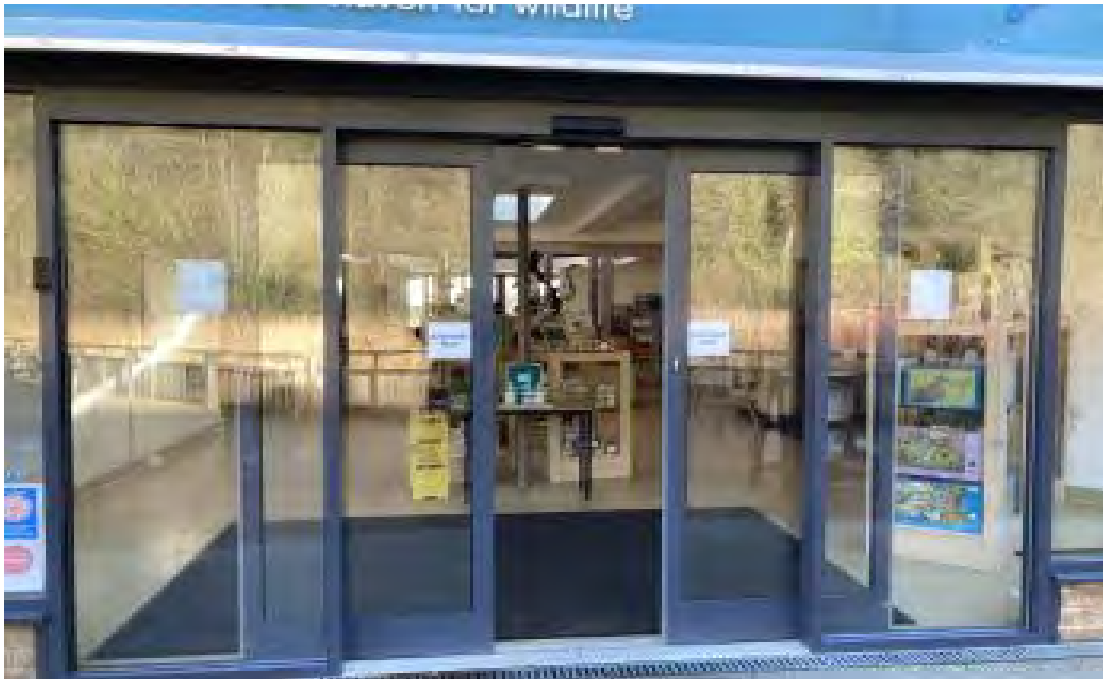
This is the entrance to the Visitor Centre Automatic with sliding entry doors
